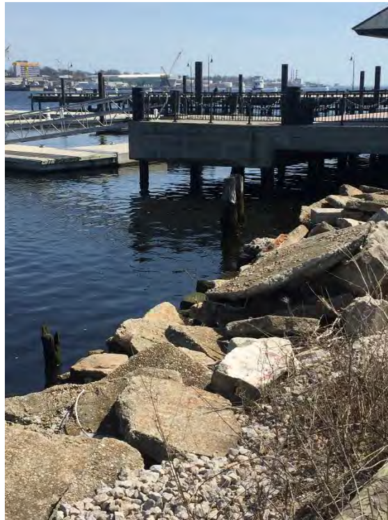
Existing Conditions: View of City Pier overhang from Site
