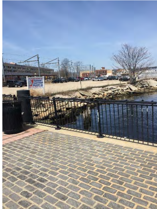
Existing Conditions: View of Site from South and East
