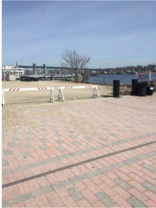
Existing Conditions: View of Site from South and West
